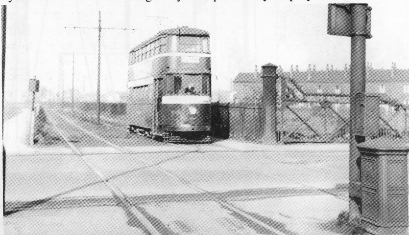
The new shed site on 26th March 1959. Feltham No.526 slows to cross Burton Road, the driver looking warily for approaching road vehicles. The tram rails immediately in front of the photographer have just been lifted to enable track to the shed to be laid in. Photo: J.A. Peden.
