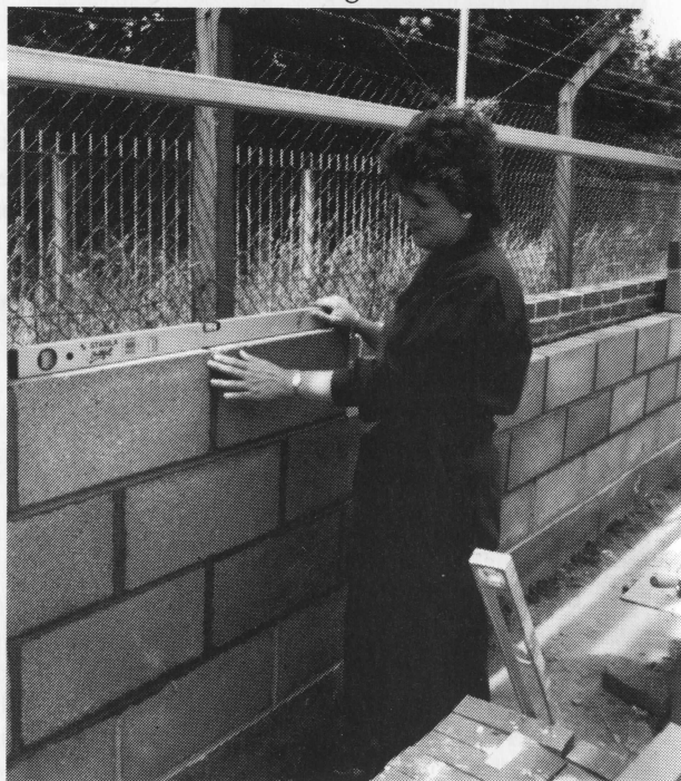
Karina Smith checks her own (very creditable) handiwork on the breeze-block lining of the new shed's west wall. Photo: Stan Holdsworth
