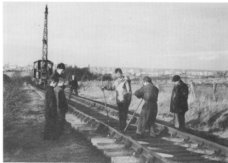
Above: 'slewing' the newly laid track. Below: lowering in the last new panel.
