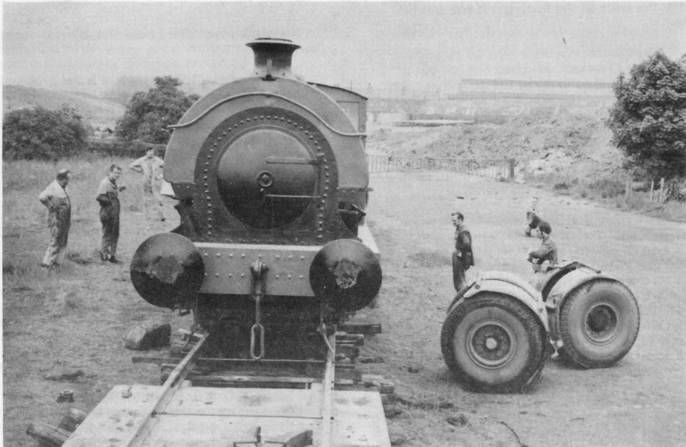
Arrival — No 6 is unloaded on June 5th 1971, after its journey from Swanscombe, on to the headshunt, which has since been lifted in connection with the realignment project. (Photo by John Edwards)
