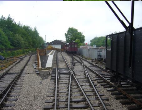
Driver's eye-view of the approach to Moor Road station with the passenger coaches standing in the run-round loop service for the next day's service and ex-NER goods brake van in Bannister's siding
