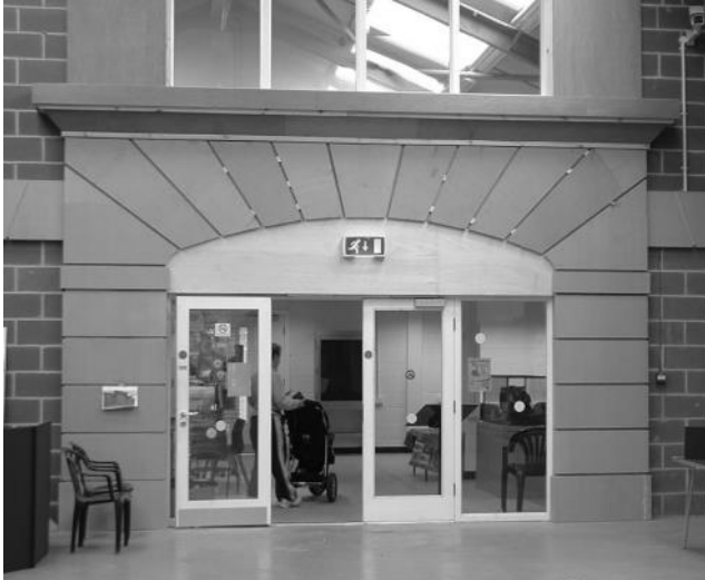
The Kitson Arch, referred to in this article, in its final stages of construction, on 9 July 2006. This view taken from inside the display hall and looking into introductory gallery and cafeteria. (Andrew Gill)
