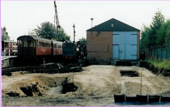
View of the site of the New Workshops, showing the footings being excavated in 1995
