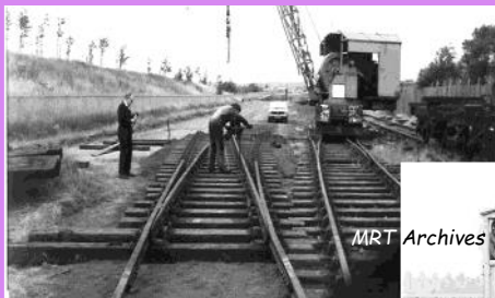
Moor Road yard from the south, showing track laying in progress in the early 1980s
