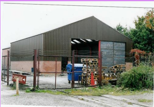
Brickwork and external cladding has been added and the end doors are being fitted
