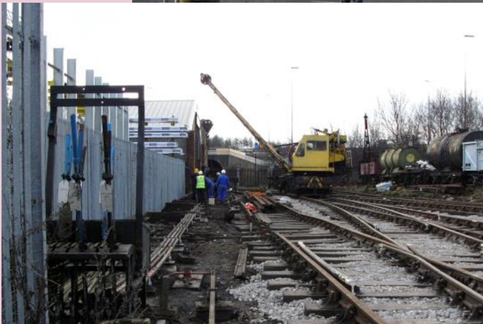
Trackwork and point rodding being finished off in Bannister's siding with assistance from the ex-British Steel Scunthorpe, Smiths of Rodley, Leeds crane
