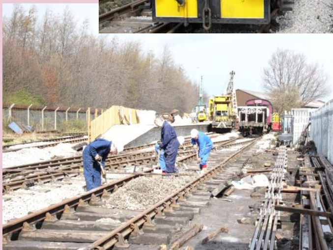
On 1 April 2006, final touches are made to the last length of track to be laid, completing the new track layout. Point rodding is complete and the visit of HM Railway Inspectorate is due in two days' time
