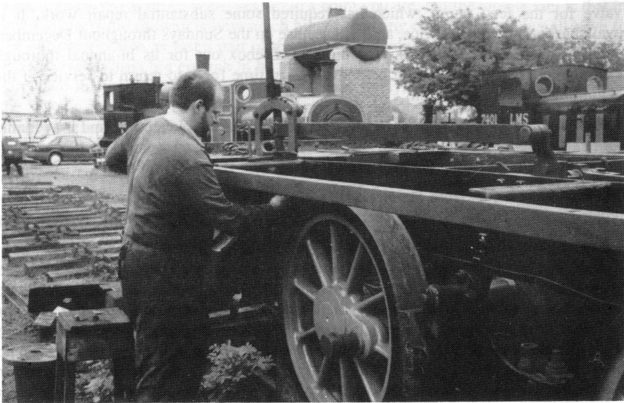
Derek Hirst adjusting the Y7's gear mechanism - again, a good chance to see parts that normal gricing doesn't reach (at least, not without a great deal of trouble and mess). Photo: Steve Roberts.
