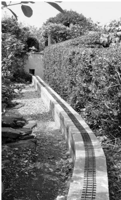
Track is laid before ballasting
