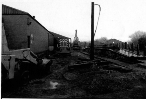
The scene on 14 April 2005. The loco pit is being filled, and the track has been torn up in the Moor Road loop prior to the new link road (see photo page 28) being installed from the back road to give access to the workshop and car park. The station platform is in course of being dismantled. (HWB)
