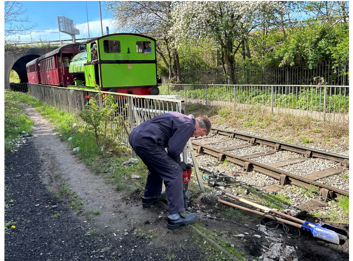
Bannisters crossing, showing (left) the new signs and (right) John Blakeley breaking out concrete for the new section of fence.
