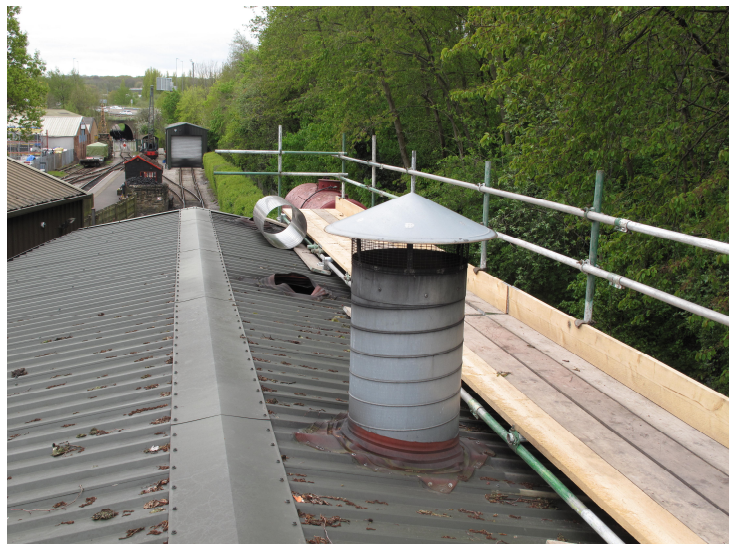
The running shed roof, showing (from far to near) one of the new smoke vents ready for fitting, the hole where one of the old vents has been removed, and another of the old vents still in position.
