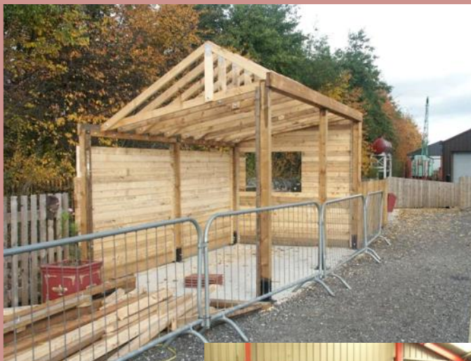
Left: The coaling stage has been completed and the passenger shelter is well under way on the platform at Moor Road. When completed the shelter will have wooden sides and a tiled roof. 3 November 2007
