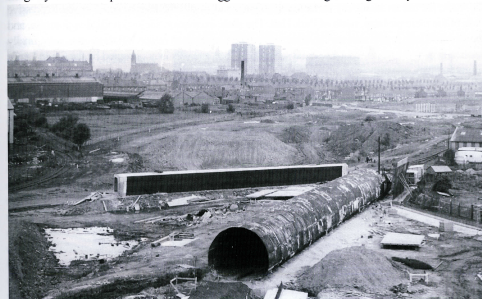
The pedestrian and railway tunnel shells await the building of the motorway embankment, 1971
