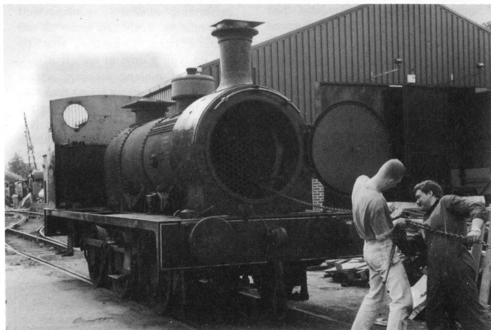
Courage , with a little help from her friends, draws the old tubes from 67's boiler, in September 1996. Photos: Graham Smith
