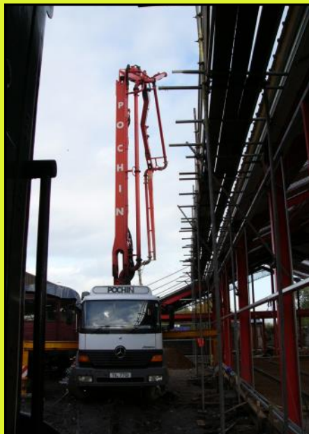
ABOVE: Pouring concrete into the base of the Exhibition Hall (HWB)
