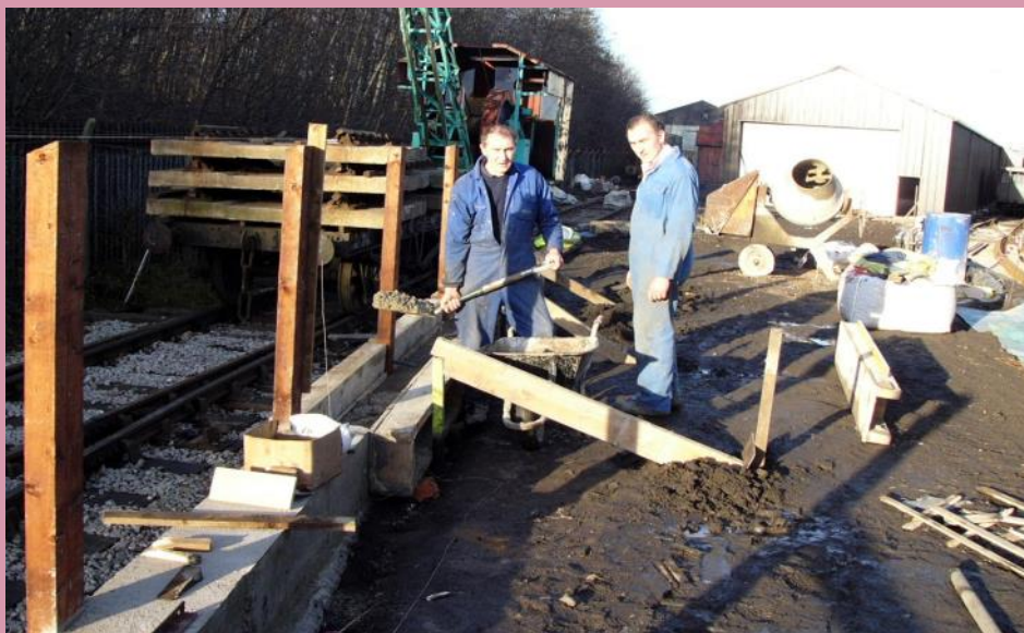
ABOVE: 25 January 2006, and Neil and Phil Carmichael are pouring concrete into the formers at the rear of the new platform (HWB)
