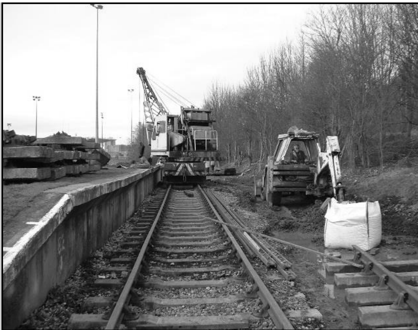
On 20 January 2008. TOP: the run round loop is removed and the trackbed is being lowered to accommodate concrete sleepers. BOTTOM: New platform extension blocks in place, and the end slope being craned back into position. (Andrew Gill)
