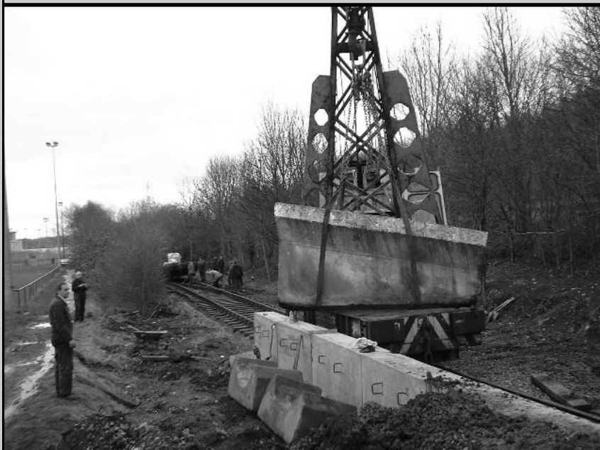
On 20 January 2008. TOP: the run round loop is removed and the trackbed is being lowered to accommodate concrete sleepers. BOTTOM: New platform extension blocks in place, and the end slope being craned back into position. (Andrew Gill)
