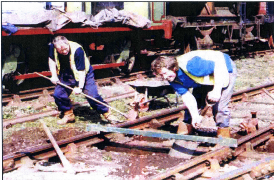
ABOVE The Father and Son team of Brian & Lee Hall are busy with a spot of jacking and packing on the loop at Moor Road.
