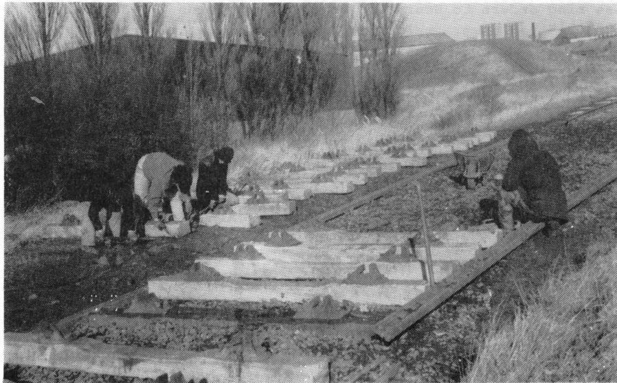
Above: recovery of rodding at Normanton, September 1987. Below: laying concrete sleepers south of the tunnel. Both described in the Spring issue. Photos: S.J. Roberts.
