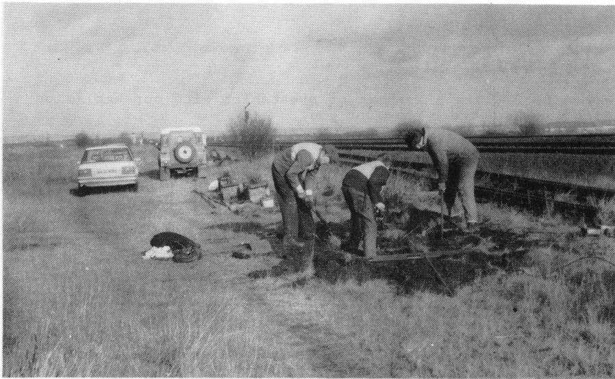
Above: recovery of rodding at Normanton, September 1987.
