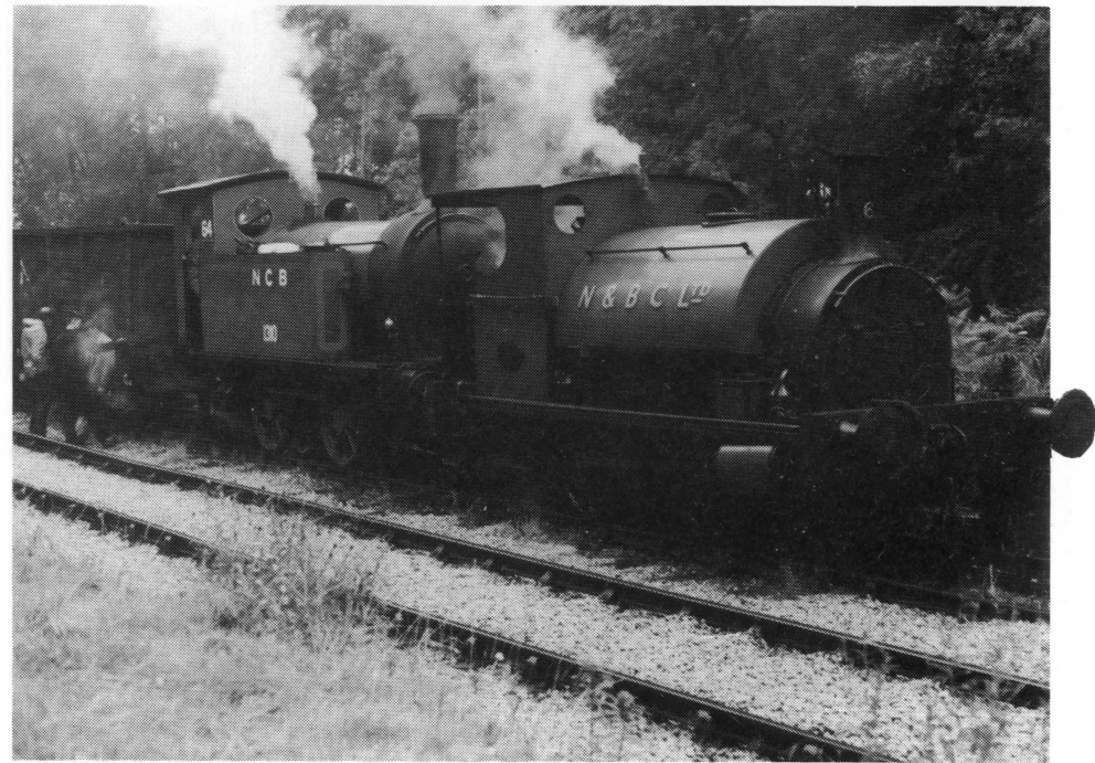
1310 pictured at Dilhorne Park, double-heading a demonstration freight train with the Robert Heath 0-4-0ST No.6, which was built in 1886. The photographer's father mentioned that "Rumour has it that the locos were coupled the opposite way round at first but, with No.6 being so much smaller than 1310, the crew of the latter felt a bit uncomfortable with its exhaust whistling past their ears!" Photo: Andrew Plumb
