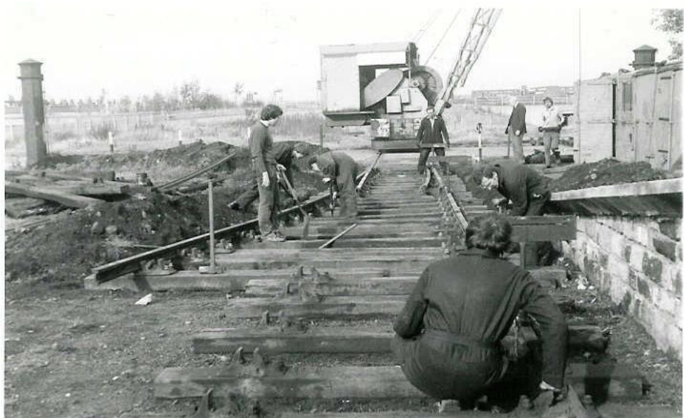
October 1982 — Our first station under construction. Laying the turnout to form the run-round loop at Tunstall Road, later Moor Road, terminus. (Steve Roberts)
