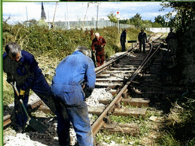
Spreading and packing of ballast continues apace , with level boards in position, to ensure a smooth ride for the All Line Tour trains at the September Gala weekend. 30 August 2003 (HWP)
