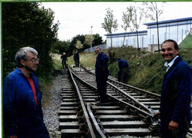
Final day's work after several weekends of labour, and following the delivery of the ballast by the Dogfish ballast wagon: levelling and packing the turn-out on the Balm Road branch after relaying, making ready for the Gala weekend. 30 August 2003. (HWP)
