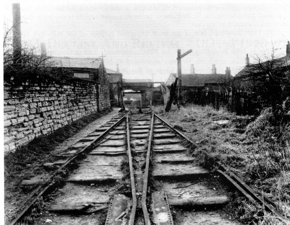
Looking south up the top end of 'Rope Hill', the upper incline, in November 1950. Note the simple wooden signal, right, and the sloping retaining rollers for the wires. Photo: Leeds City Engineers, reproduced by kind permission of Leeds Reference Library.
