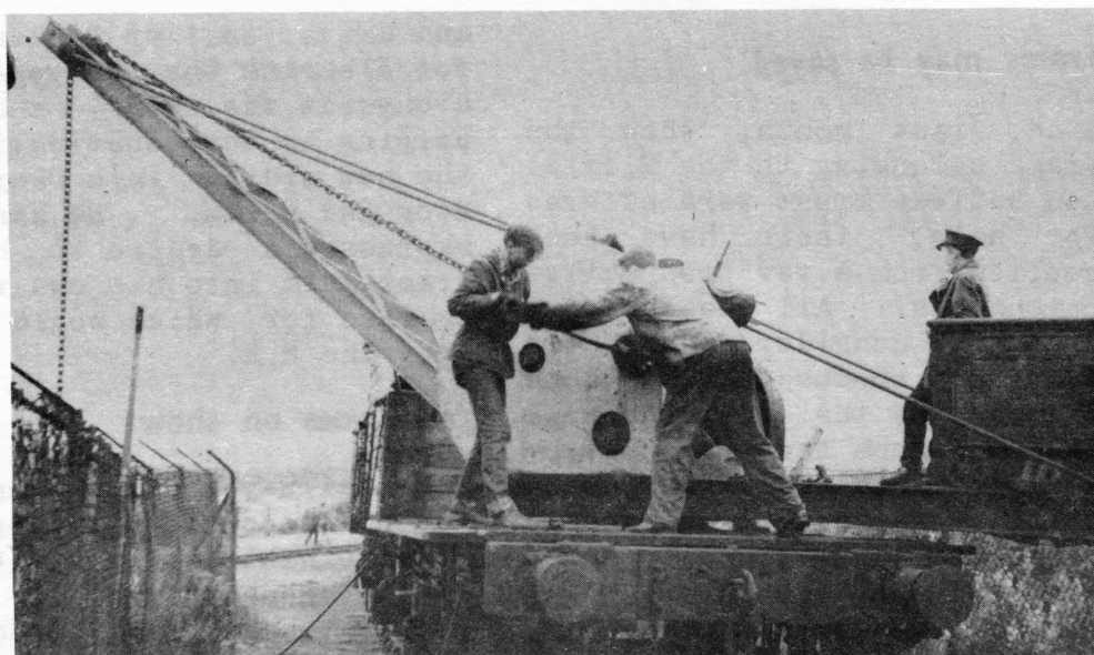
The 1888 Midland Railway hand crane has recently been restored to working condition, and is seen here being tested at the foot of Clayton's curve.
