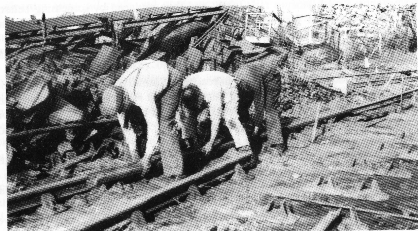
A 1971 p.w. gang at work re-aligning R.&B.'s turnout. Photo: John Edwards.
