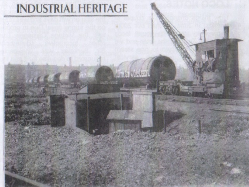
Below Ltd shows crane shunting a long rake of railway wagons loaded with Lancashire boilers built by Clayton, Son & Co Ltd, Leeds.
